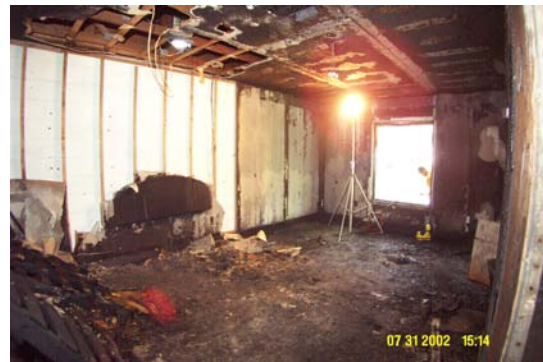
Figure 6 – Fire room looking from entry/exit towards window
