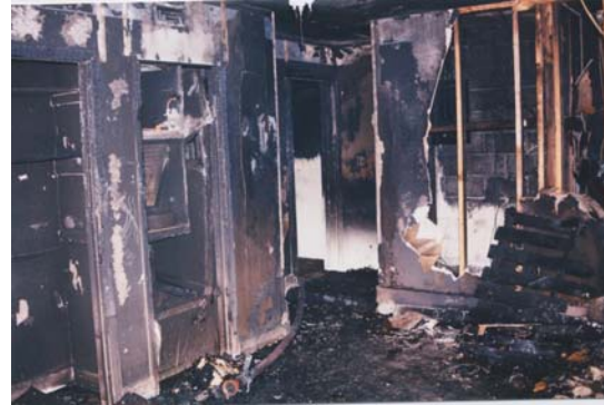
Figure 5 - fire room from corner opposite of entry/exit
